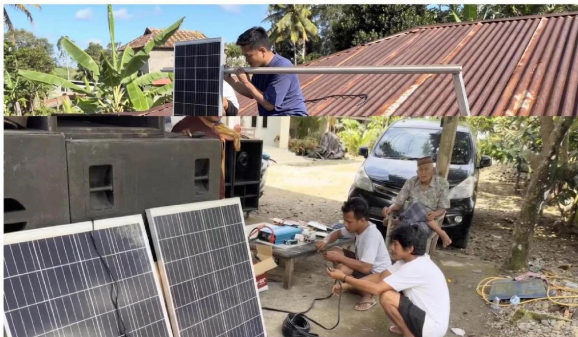
Figure 1. Installation of the solar photovoltaic system and hybrid incubator at the partner site (June 2026).
