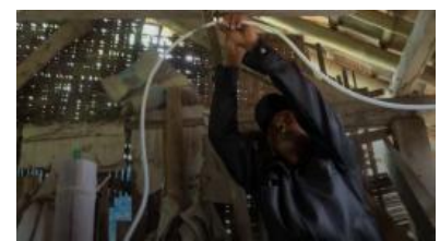
(c) pemasangan misting nozzle
