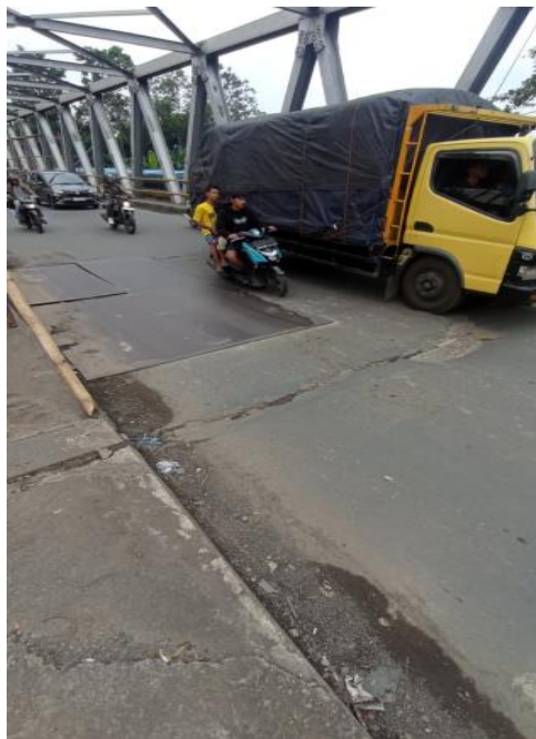
Figure 1. Documented condition of the existing reinforced concrete bridge deck.
